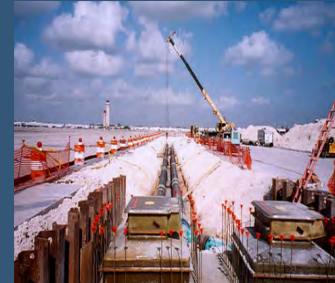
Installation of AHS piping and vaults
